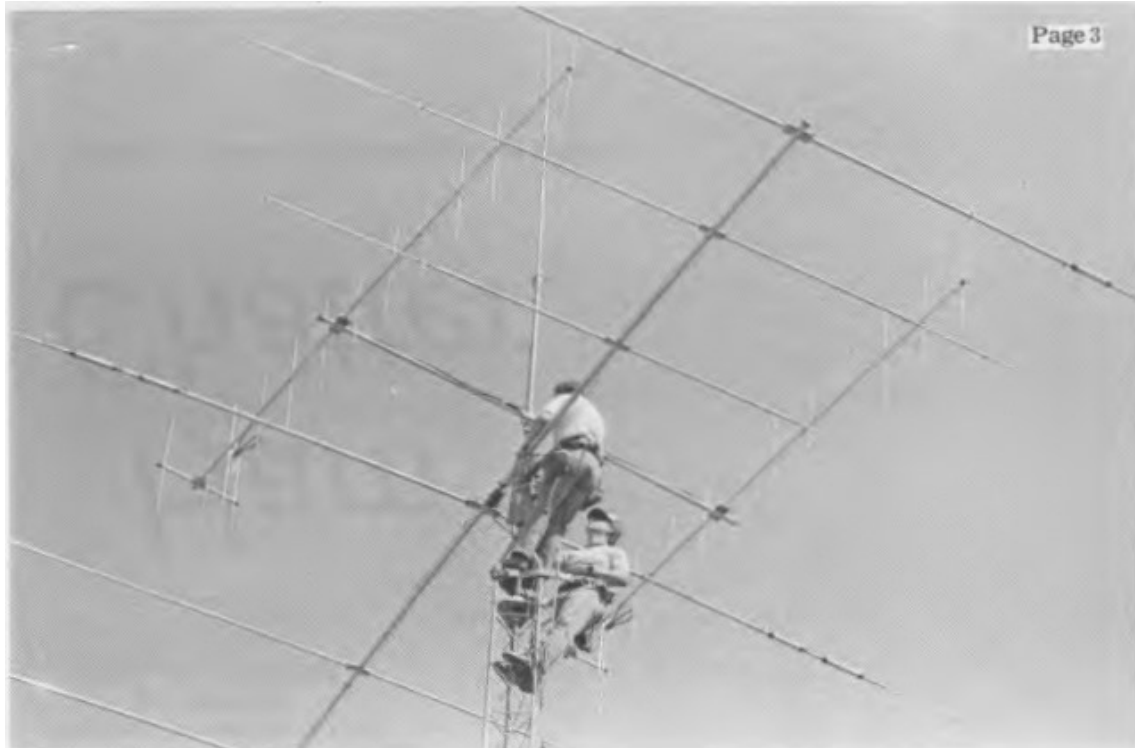
ANTENNA ART? . . . Burnie Nobles and Donnie Hudson make final adjustments to a double stacked "Boomer Jr." array on Donnie's tower recently. The results of the system were not
